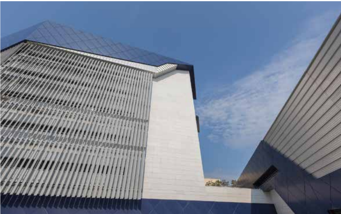
Precast material was used for cladding the Life Sciences building as well.
