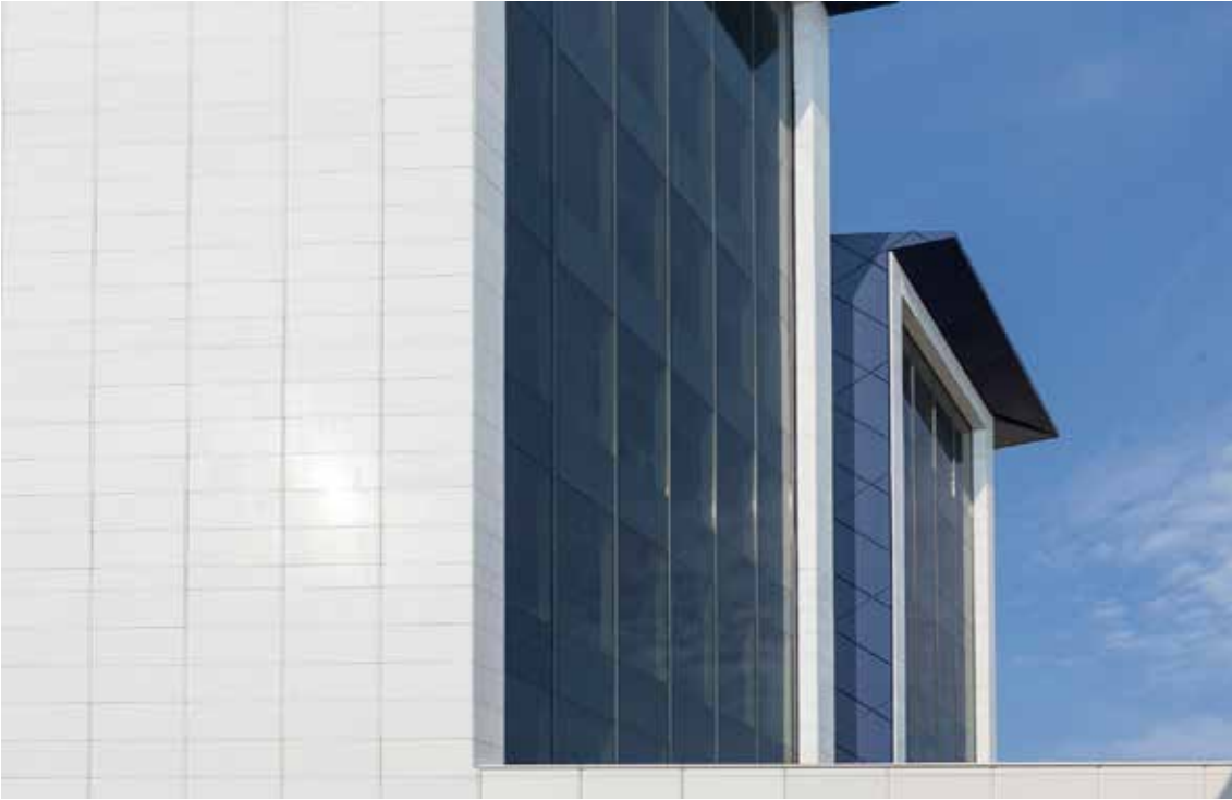
Precast material was used for cladding the Life Sciences building as well.
